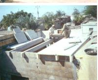
This load bearing construction is 1/3rd the cost of RCC (Reinforced Concrete Construction).
