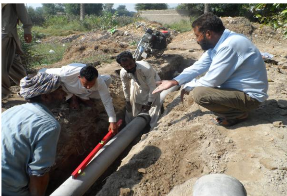
PWO- Harand, South Punjab Supervision of the first lane sewer being laid in Chah Baloch Wala
