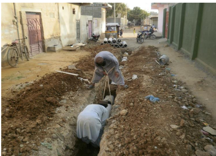
A lane sewer being laid in Gulshan-e-Behar, Orangi Town supervised by OPP-RTI's team
